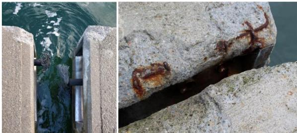
**Figure 2.** Breaking of the connectors and damage on the concrete modules.
