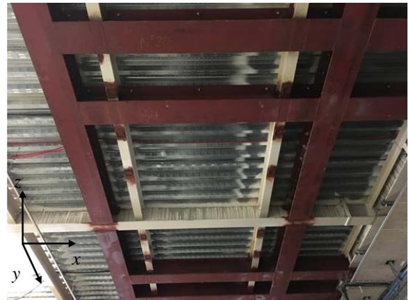
**Figure 8:** Added steel beams (dark red) to strengthen the slab
