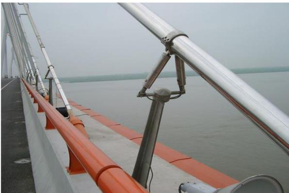
**Figure 11:** Dongting Lake bridge. Assembly of the dampers <sup>[20]</sup>.
