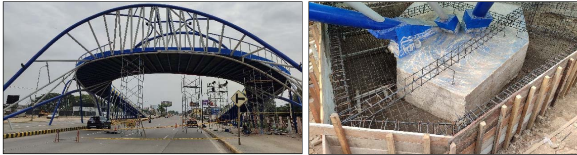
Figure 6: Reinforcement of arches and bridge foundation
