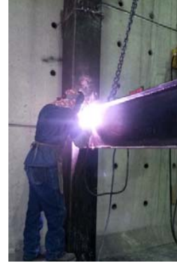
Figure 3. Welding of the connection.
